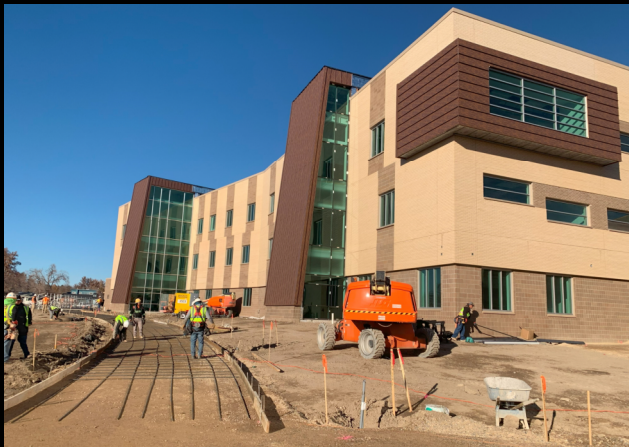
Metal Siding & Site Concrete Prep
