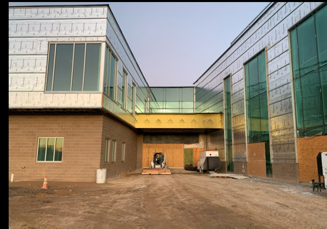
Exterior Glazing and Insulation
